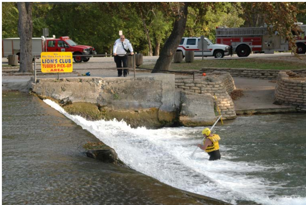
Lt. Kelly Metz probes the base of Rio Vista Dam in the heavy current assisting the consulting engineer with the evaluation of the dam.
